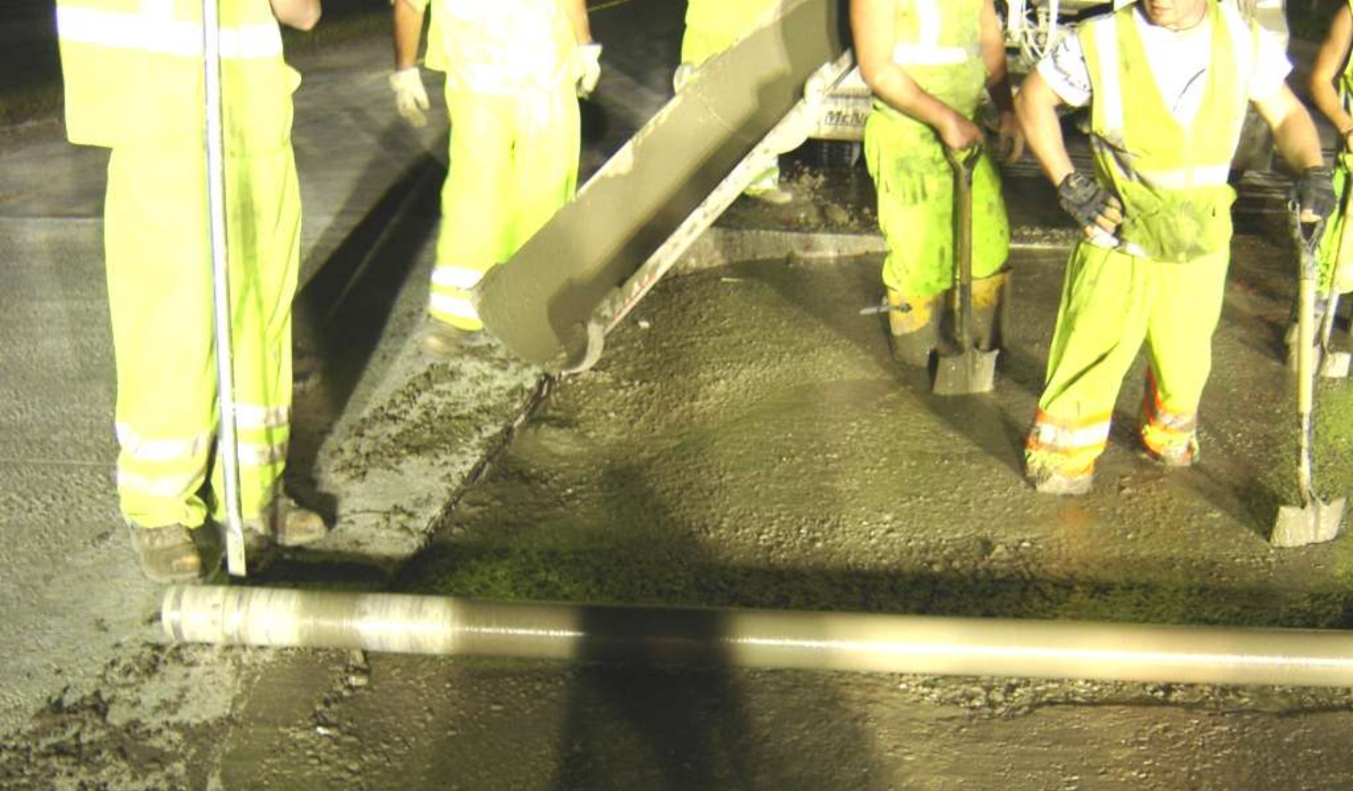
Ready Mix Truck Mixing with Roller Screed Finishing
